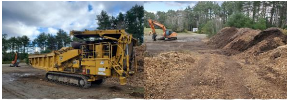
Stump and Brush pile ground up to make room for the new Highway Garage
