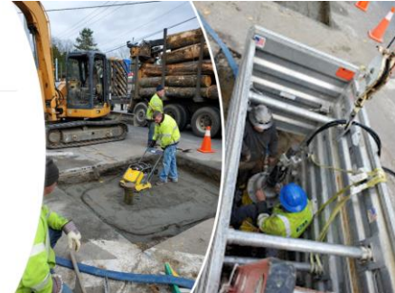
New water main valves installed at the Bank and at Dynamite Hill
