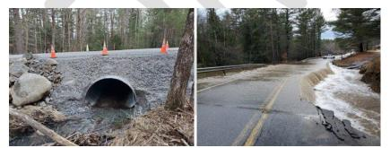
Hidden Lake beaver dam broke on March 20th, washing out the culvert on Hidden Lake Road and destroying the north-bound lane of County Route 19. Luckily no one was injured. The County is in the process of redesigning the culvert for this part of the road
